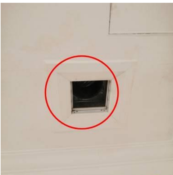
location: 1st floor Bedroom 4 bath Status: Open Comments:
