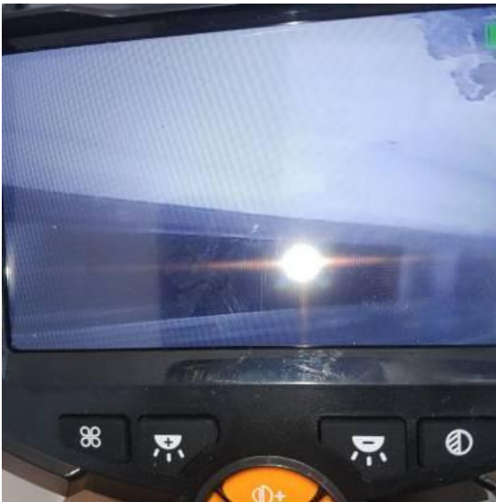
location: All AC ducts Status: Open Comments:
