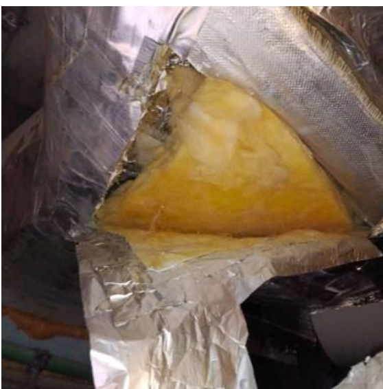
location: 1st floor Bedroom 3 Bath Status: Open Comments:
