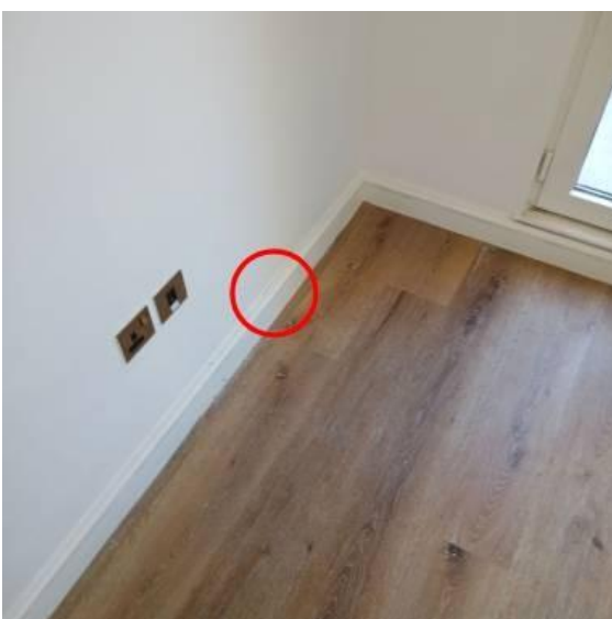
location: Dining area Status: Open Comments:
