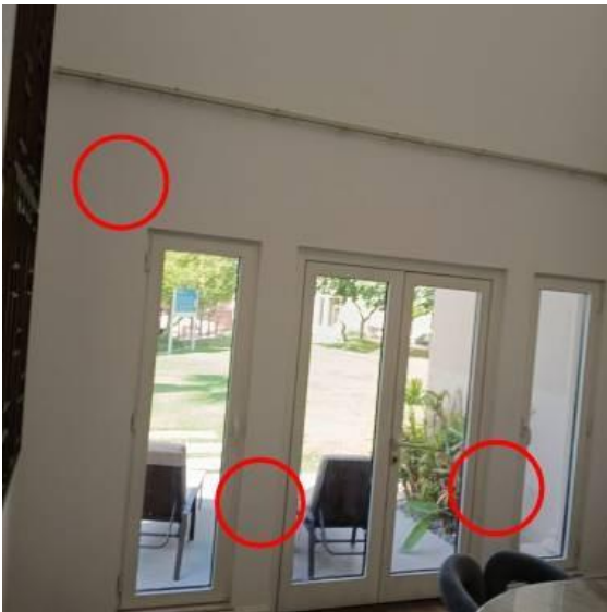
location: Dining area Status: Open Comments:
