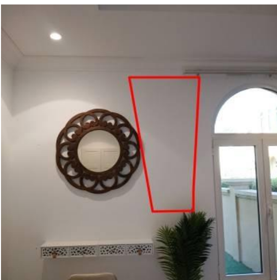
location: G.F Bedroom 1 Status: Open Comments:
