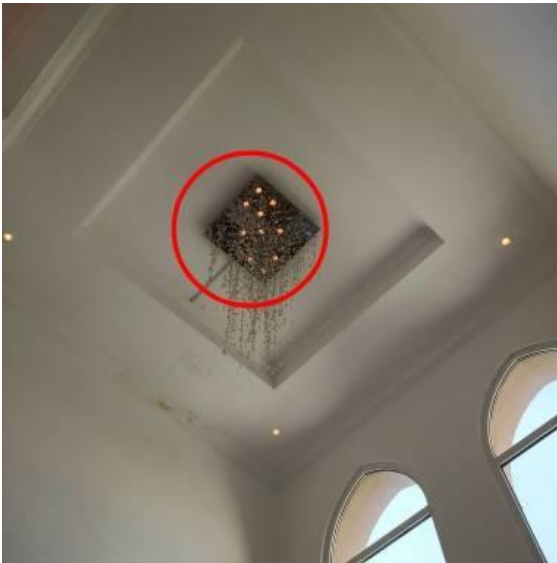
location: Dining area Status: Open Comments:
