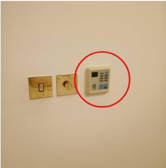
location: 1st floor Bedroom 4 Status: Open Comments:
